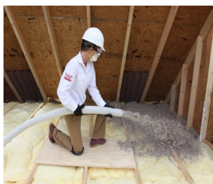
Cellulose is often sprayed over old fiberglass batts
