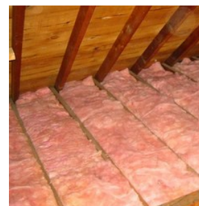
Fiberglass batts—vapor barrier correctly facing towards living space
